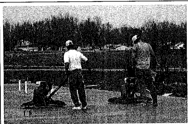
Construction at Future Hall of Fame Site St. Charles County, Missouri
